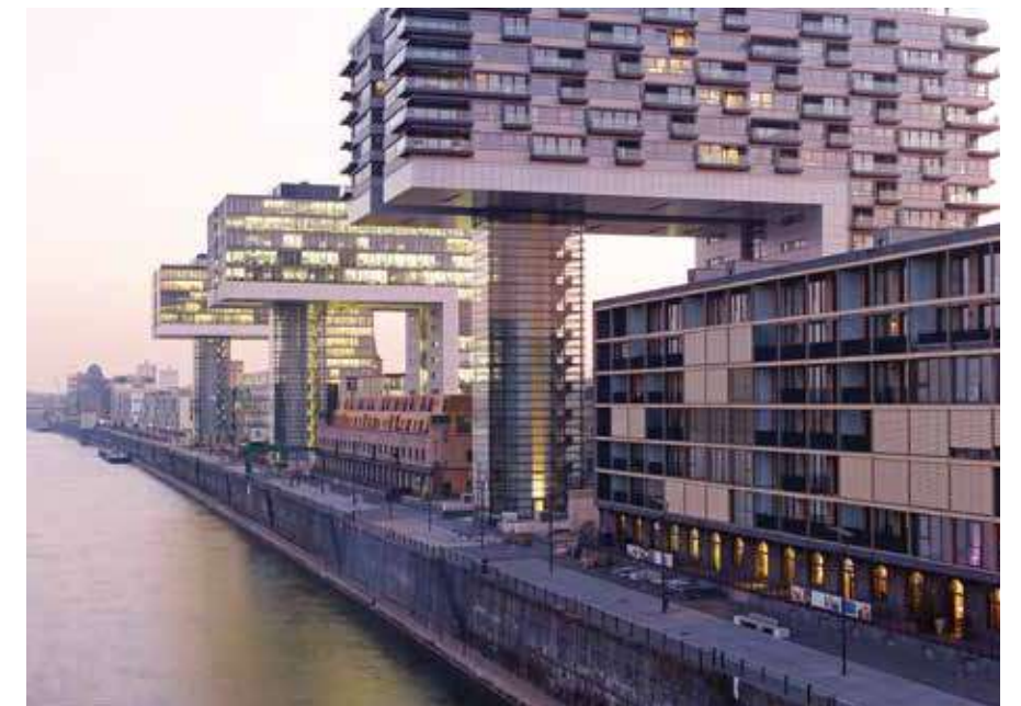
KRANHAUS IN COLOGNE, GERMANY
